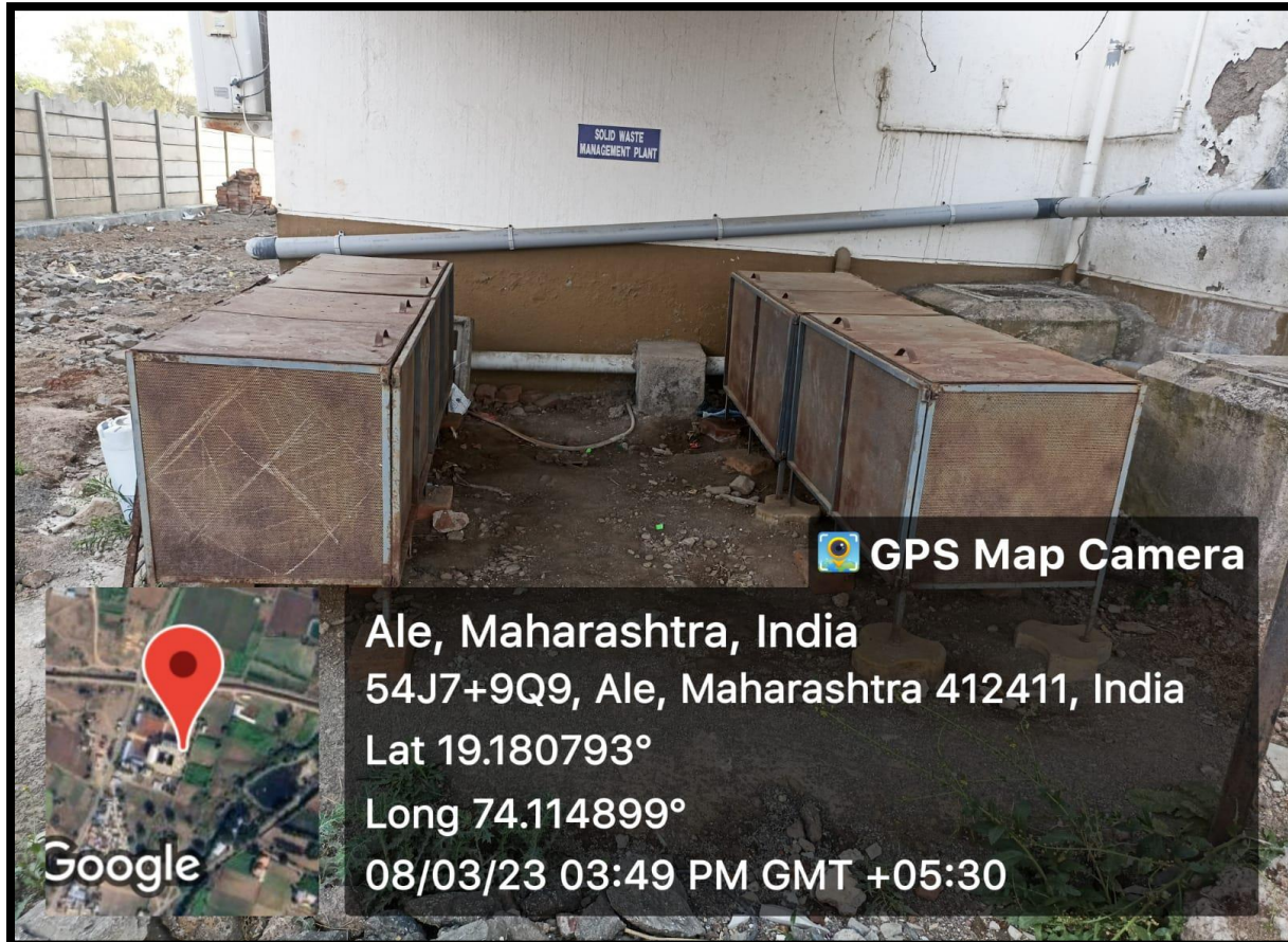
SOLID WASTE MANAGEMENT PLANT
