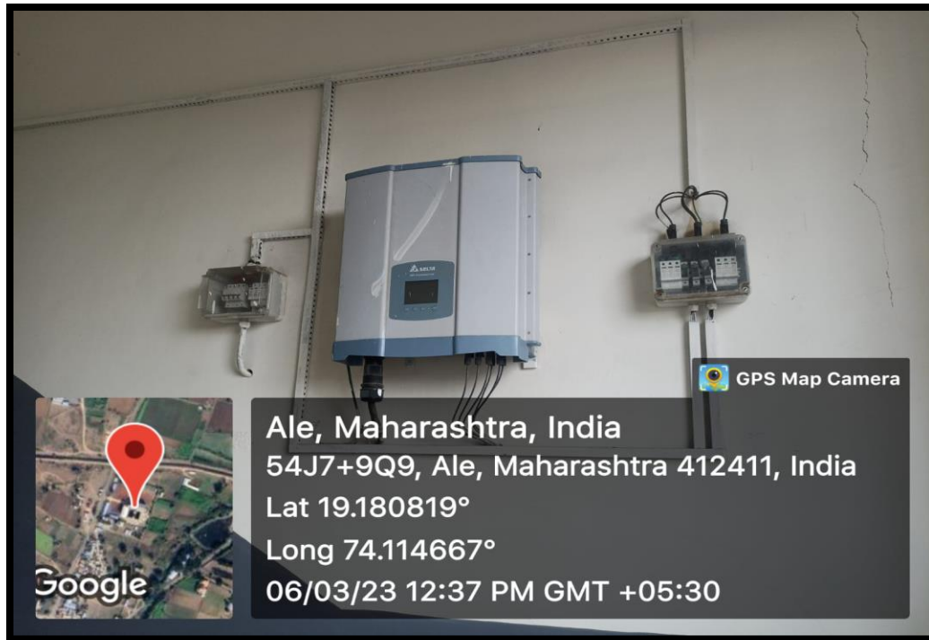
Installation of Solar System
